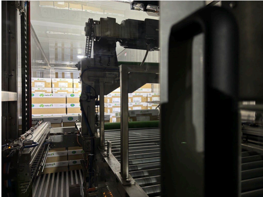
Loader in Operation
