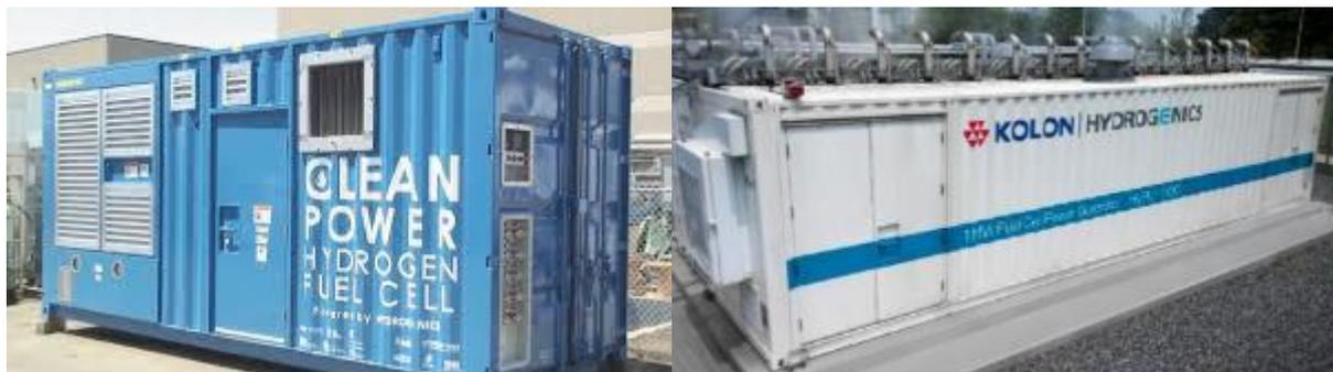
Figure 37: Containerised 200 kW and 1 MW Fuel Cell Modules with Pressurised H<sub>2</sub> Storage<sup>44</sup>
