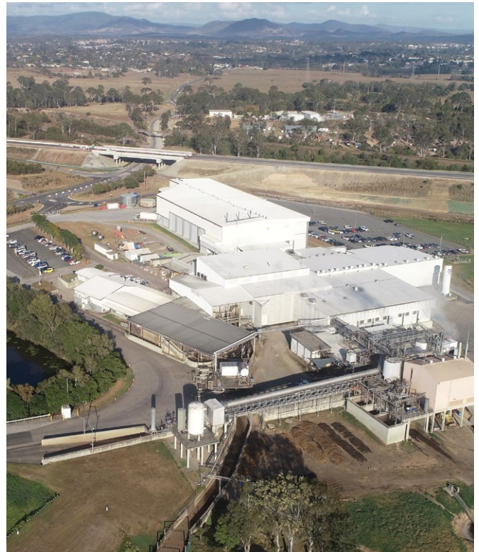
Image: Australian processing plant
