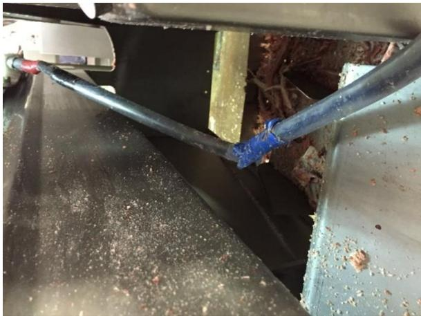
*Figure 10: Damaged electrical cable conduit*
