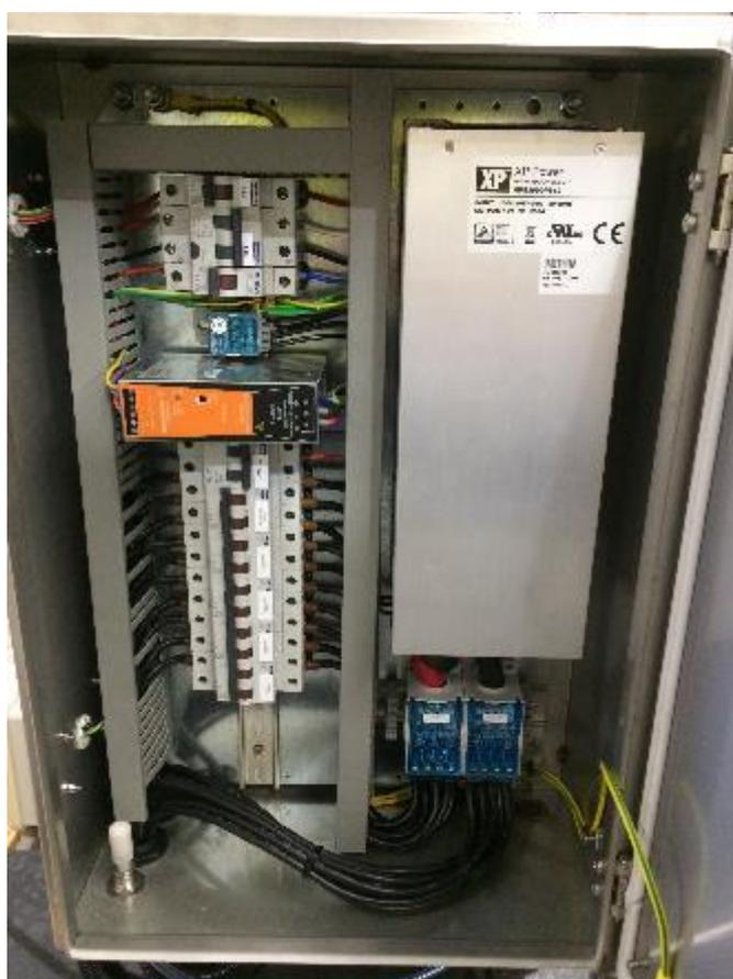
Figure 41: Electrical cabinet showing 12 VDC, 3 kW power supply, distribution blocks and safety switches.
