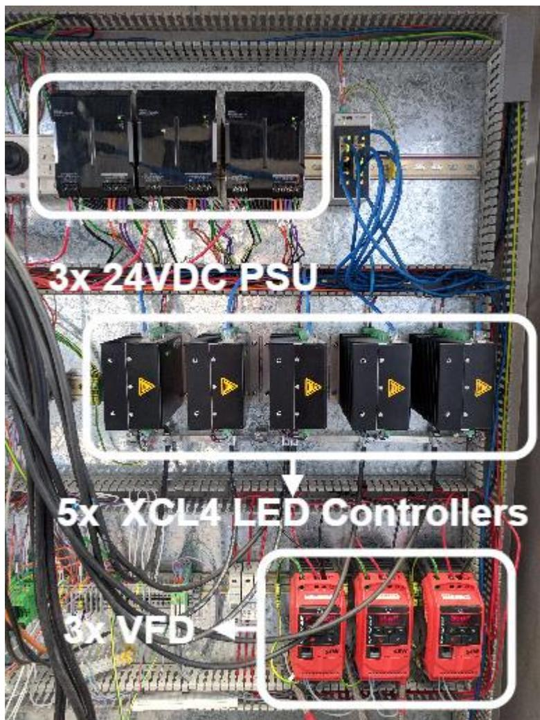
Figure 10 - Control Cabinet: PSU's, LED Controllers and VFD's
