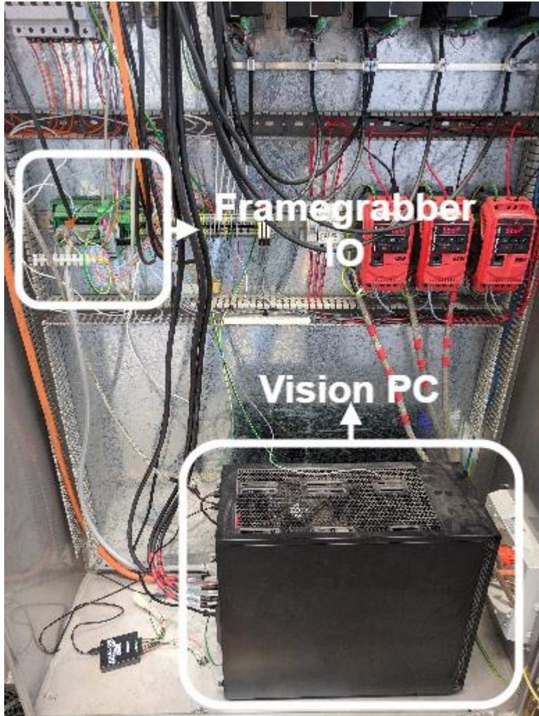
Figure 11 - Control Cabinet: Framegrabber IO and Vision PC
