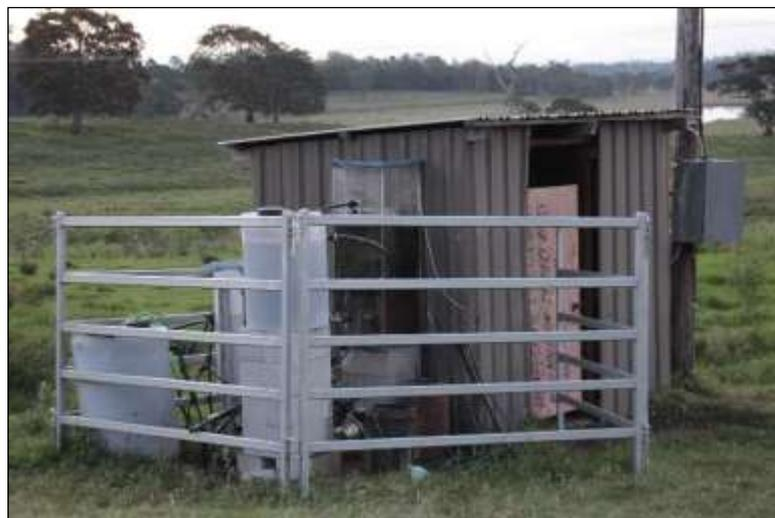
Figure 12: Struvite crystallisation plant installed at an Australian meat processor to recover phosphorous from anaerobic lagoon effluent.
