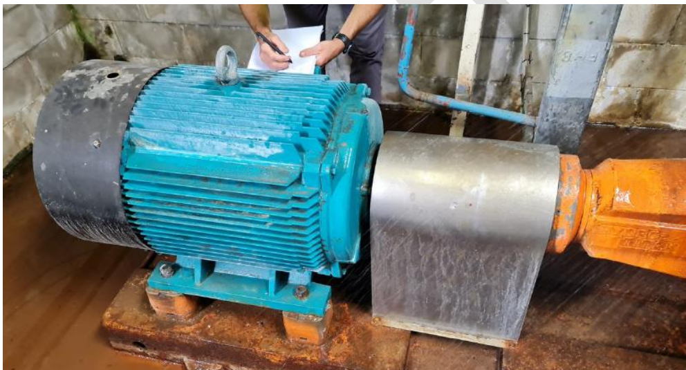
Figure 30: Old low efficiency motor being audited before upgrade at a meat works
