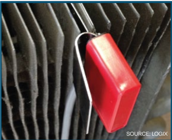
TEMPERATURE SENSOR ON EVAPORATOR
