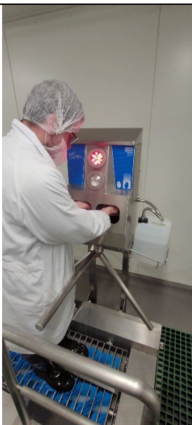
Application of both hands for sanitizer delivery ( note: red light and turnstile preventing movement until both hands are placed in receptacles)
