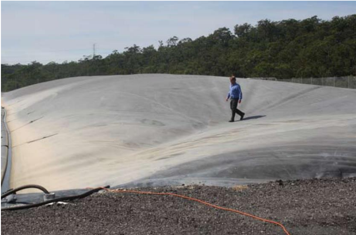
Figure 11: An example of a covered anaerobic pond (Anonymous 2010)
