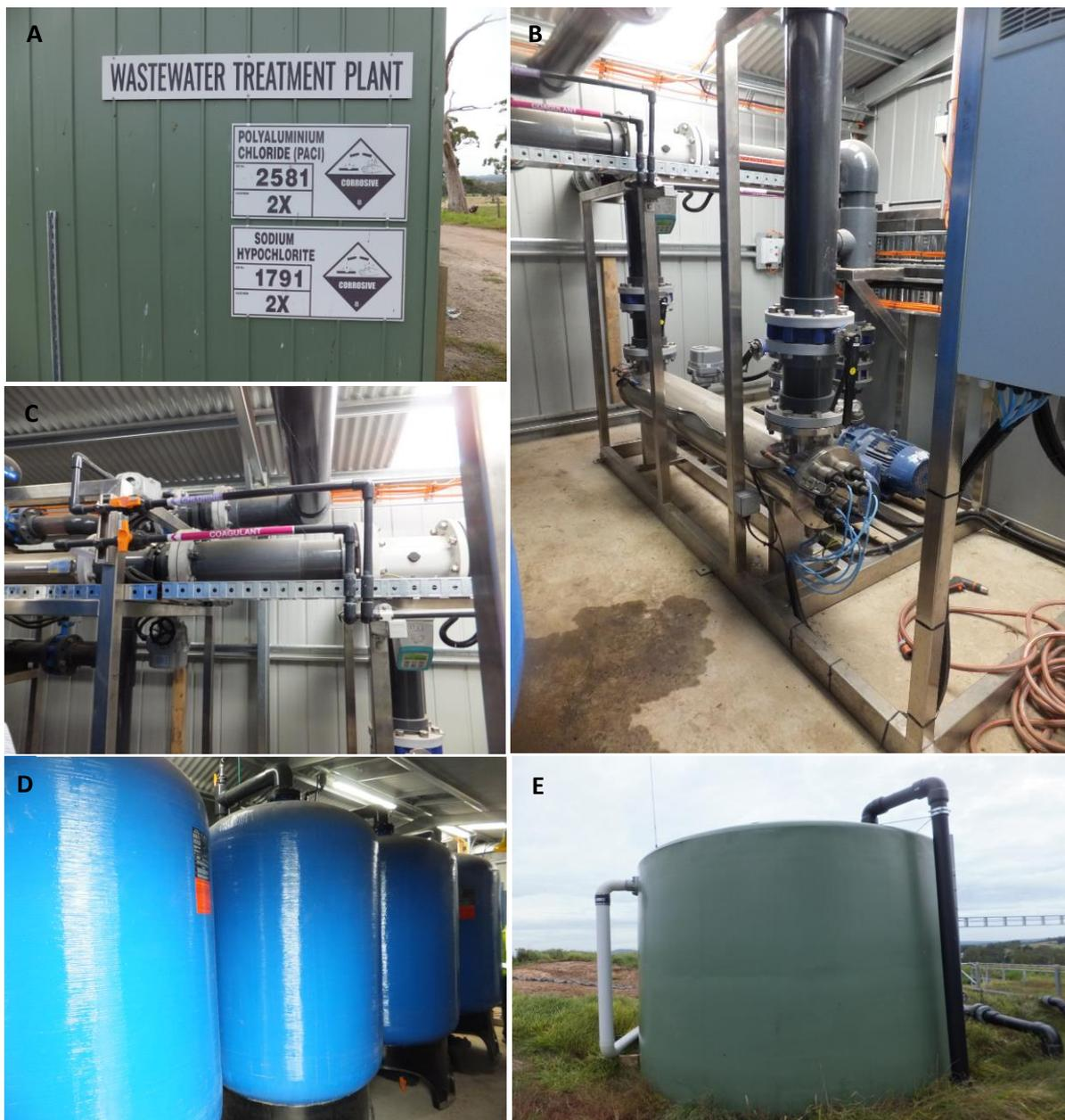
Figure 11: Wastewater treatment plant building housing polyaluminium chloride (PACL) coagulant and sodium hypochlorite disinfectant (A) for dosing into dam 6 (Figure 12), UV treatment and filtration and chemical dosing (B), UV reactor (B, centre), coagulant and disinfectant addition to raw water flow (C), four parallel flow multimedia filters (D), backflush tank for multimedia filters (E)
