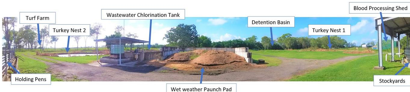
Figure 27: View and location of green wastewater stream, including Turkey nest 1,2, paunch pad, in proximity to holding pens, stockyard and blood processing shed, turf farm, detention basin and wastewater chlorination tank used for cattle yard and truck washing
