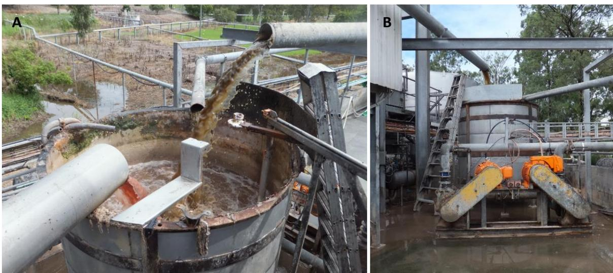
Figure 16: Saveall viewed from top (A) and ground level (B) where FOG separated red wastewater from the DAF is combined with green wastewater from the Contra shear after paunch separation
