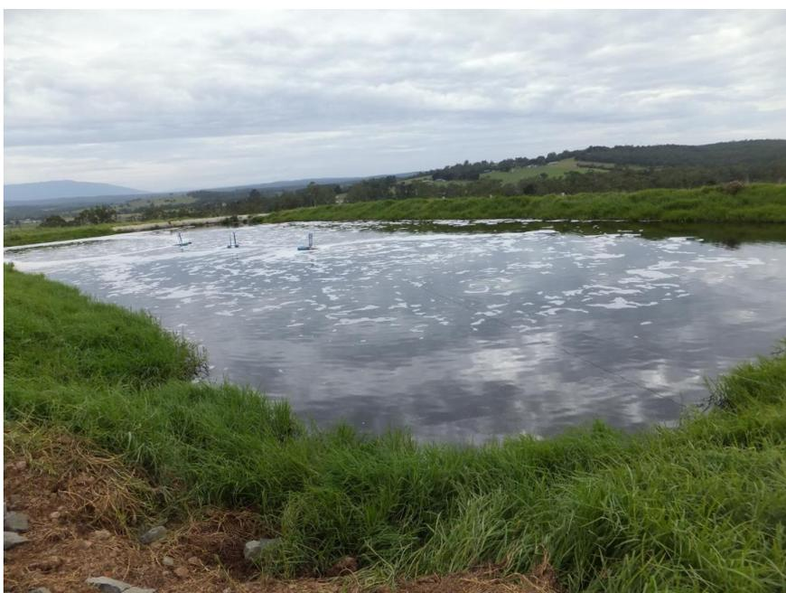
Figure 10: Non-lined dam 5 with 3 floating and submerged aerators with a total airflow of 7.2 kg/hr
