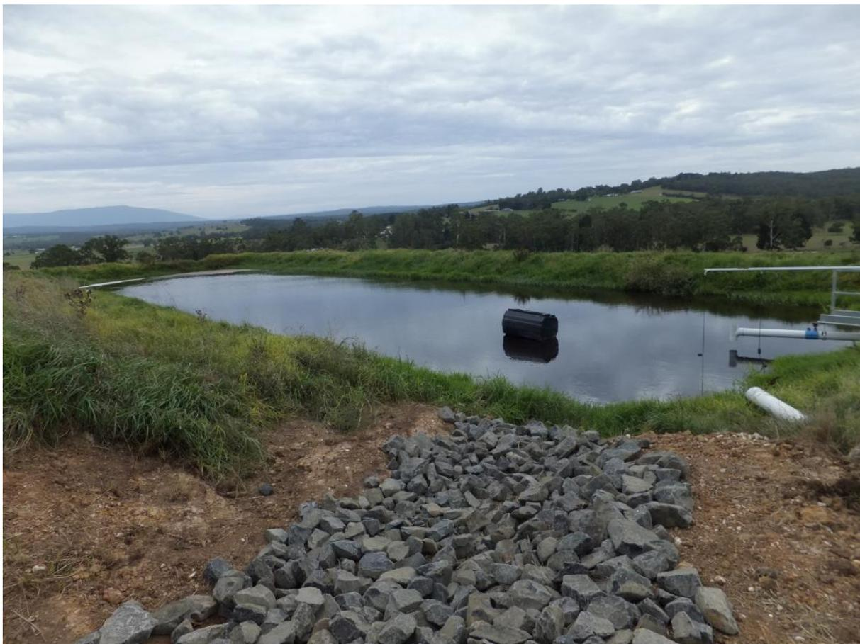
*Figure 12: Non-lined dam 6 with dosing pipes from the wastewater treatment plant (right)*
