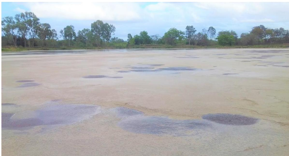
*Figure 31: Poor controlled processing with large amounts of FOG passing through the DAF-saveall pit into Dam 1*
