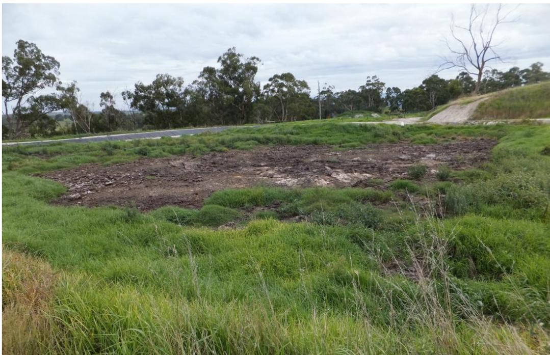
*Figure 3: Non plastic-lined earth dam 1 (pre-anaerobic pond) which receives the combined red and green wastewater from the contra shear via gravity feed pipes*
