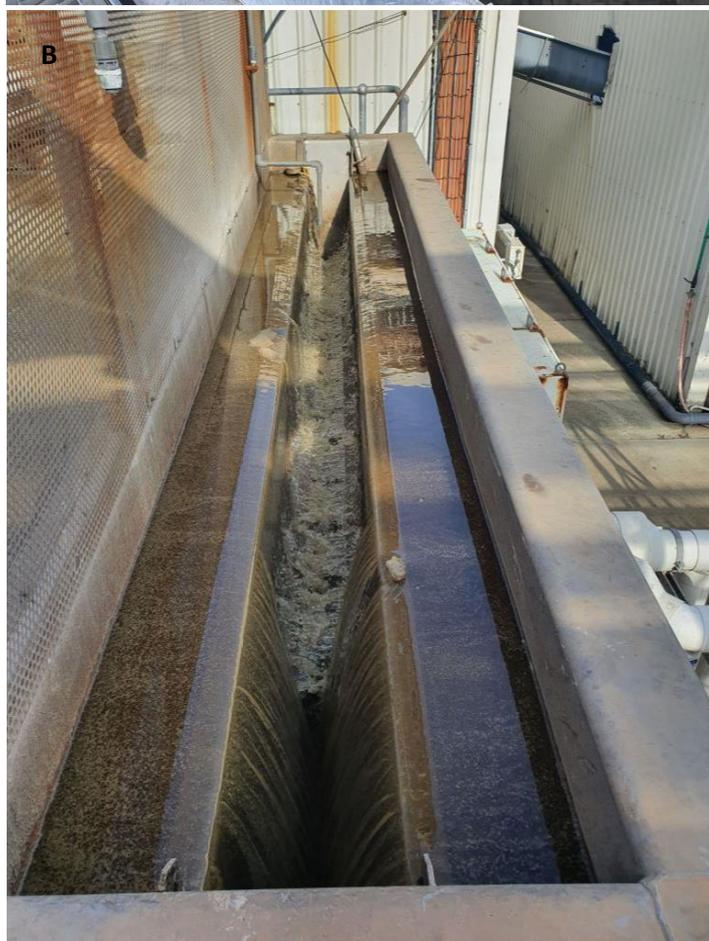
Figure 42: The surface of the DAF 2 tank showing the surface floatation sludge and chain-driven skimmers skimming the sludge into the sludge hopper (A) and separated treated water (B)
