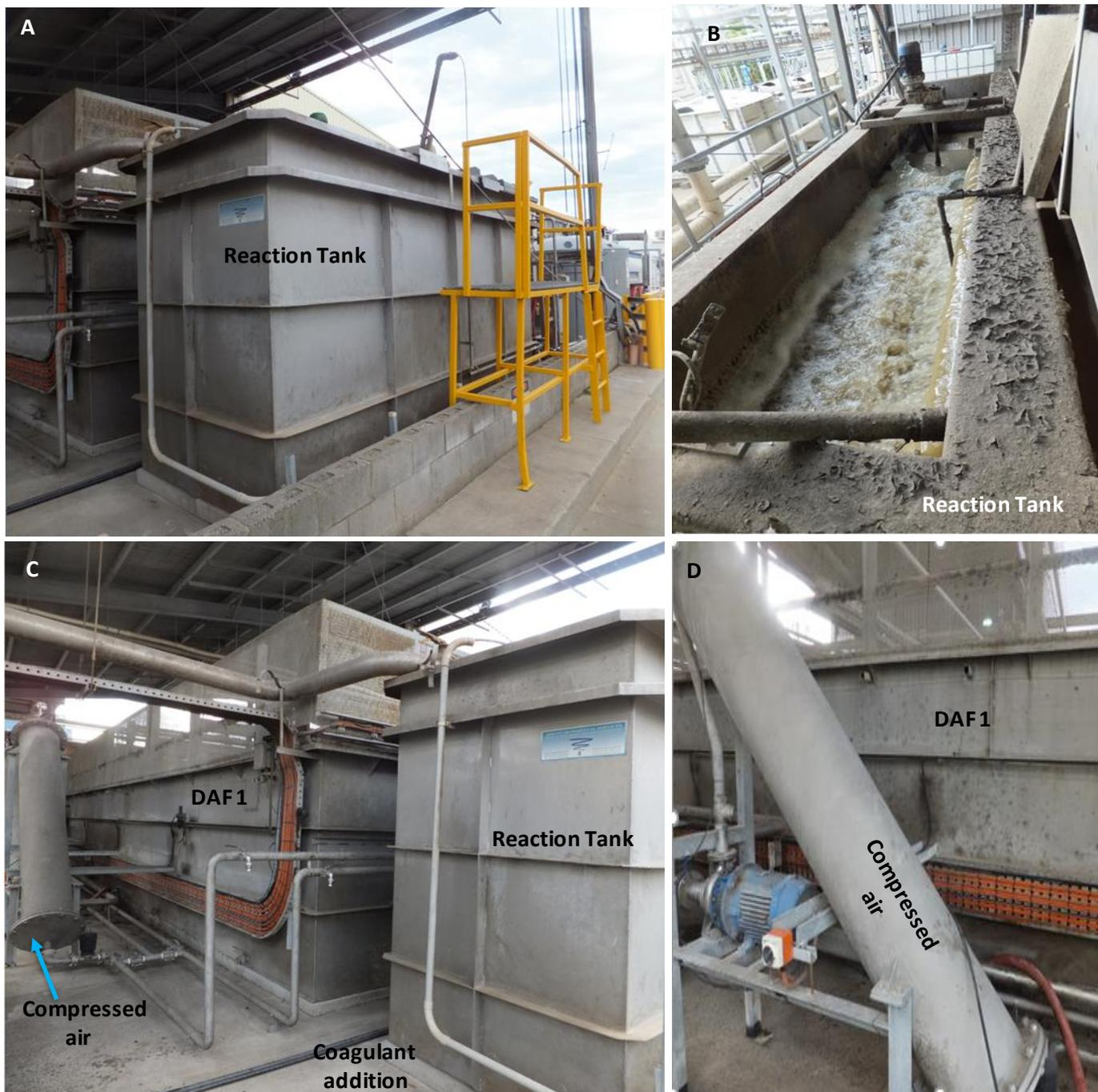
Figure 40: Reaction tank (A), inside of mixing tank (B), DAF 1 and reaction tank showing coagulant-flocculant addition and compressed air tank (C) and close-up view of compressed air tank and pump (D)
