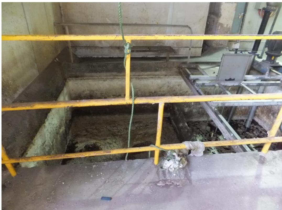
*Figure 35: Blackwater pit from rendering plant stickwater rich in fat, oil, and grease. Note the FOG crusting on the surface*
