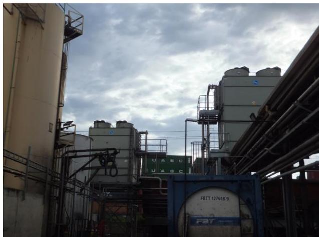
*Figure 39: Cooling towers in the background used for cooling the filtered wastewater from the buffer tank prior to going to the red tank, reaction tank, and DAF*
