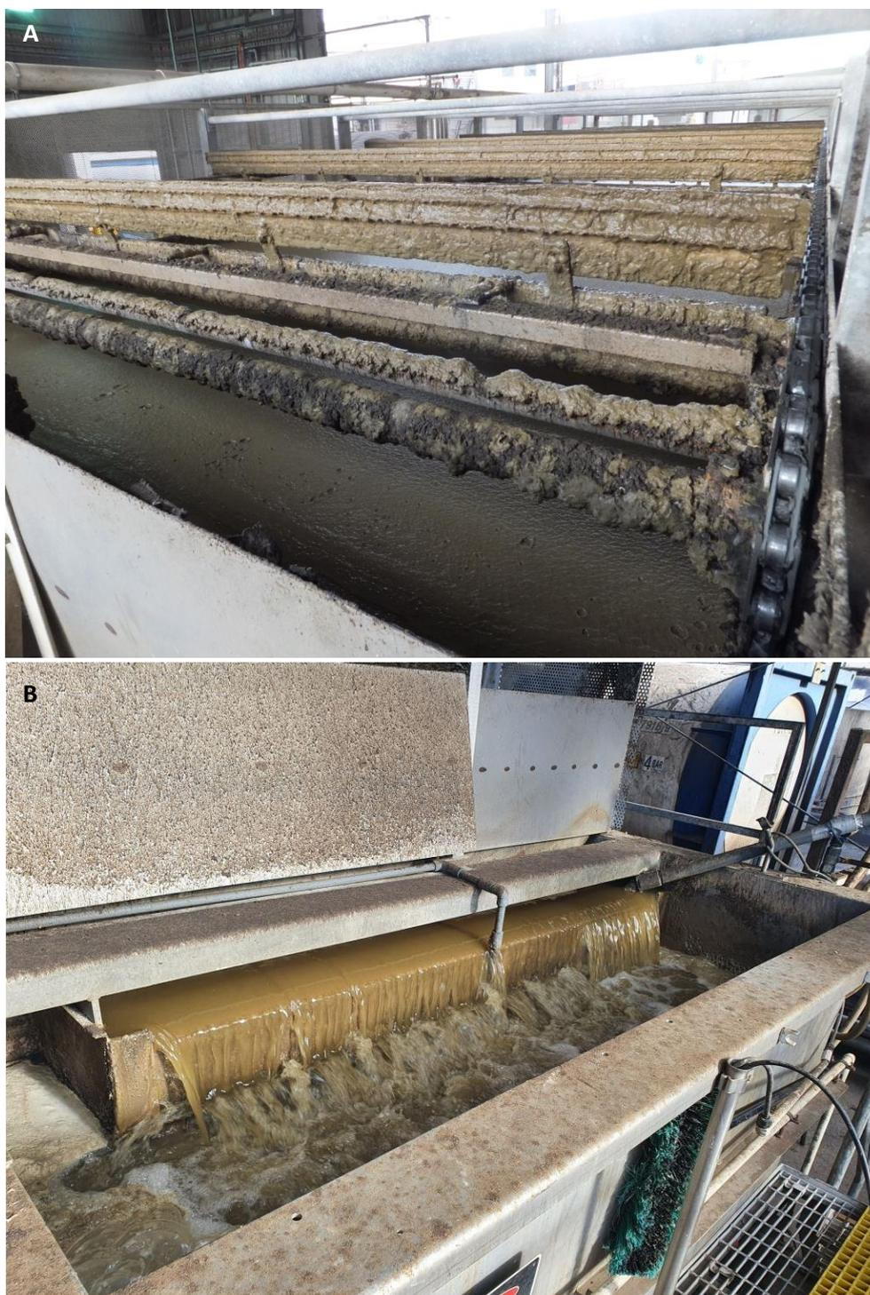
Figure 41: The surface of the DAF 1 tank showing the surface floatation sludge and chain-driven skimmers skimming the sludge into the sludge hopper (A) and separated treated water (B)
