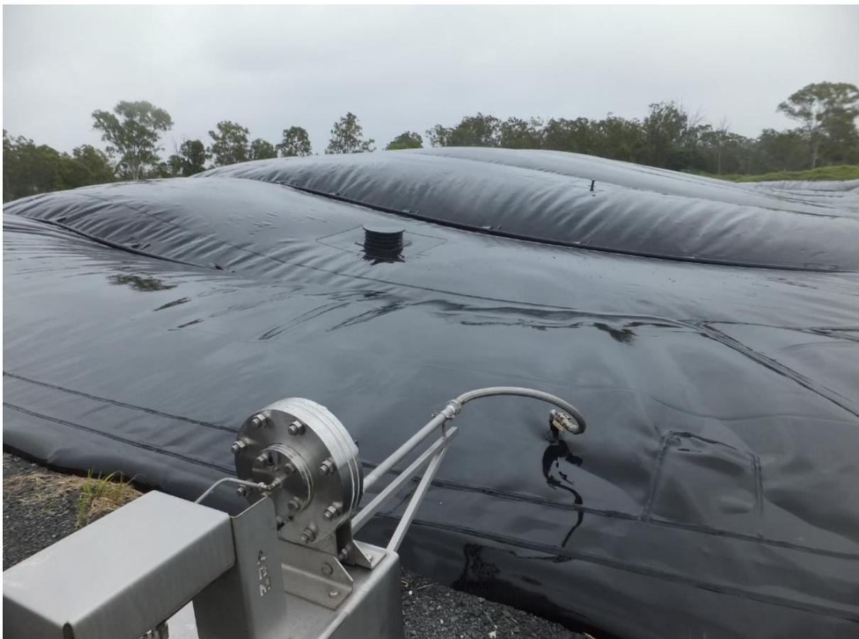
*Figure 17: Covered anaerobic lagoon (CAL) for anaerobic digestion of treated red and green wastewater from the saveall and generation of biogas collected and transferred to gas plant for drying and distribution to rendering cooker and for drying blood drier*
