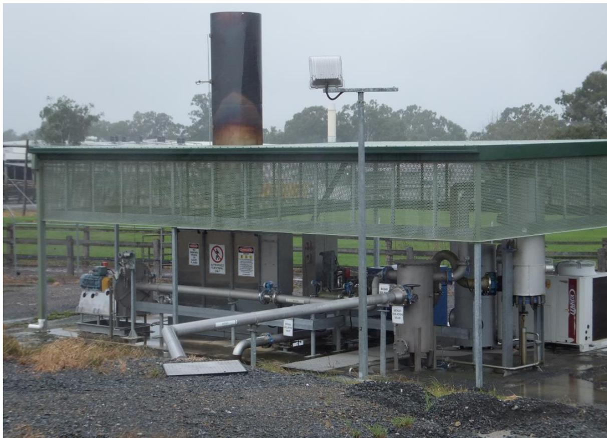
*Figure 18: Biogas from CAL (underground pipe, centre) for drying and distribution to render cooker, blood dryer with excess gas burnt at the flare stack (top)*
