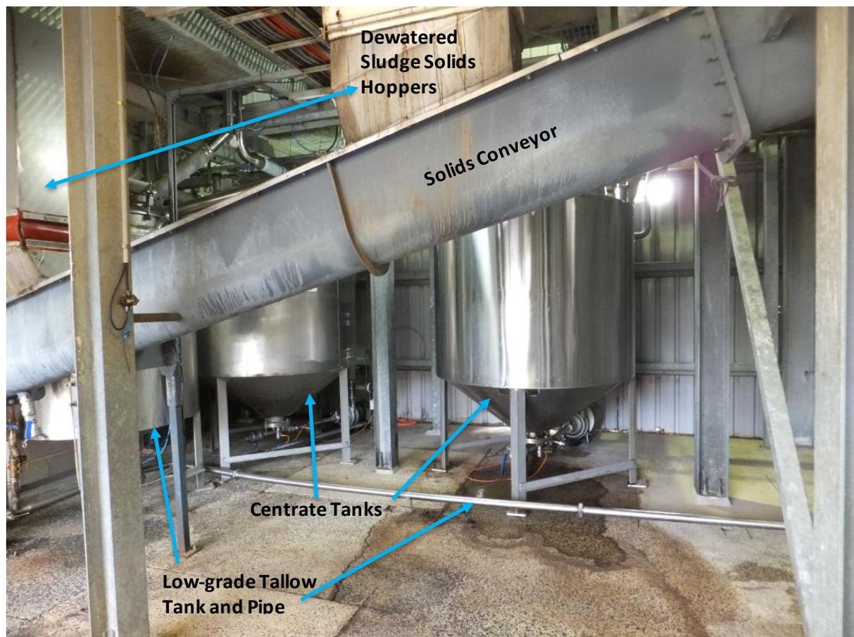
Figure 44: Centrate tanks, low-grade tallow tank (left), dewatered sludge solids hoppers and tanks conveyor to storage and removal
