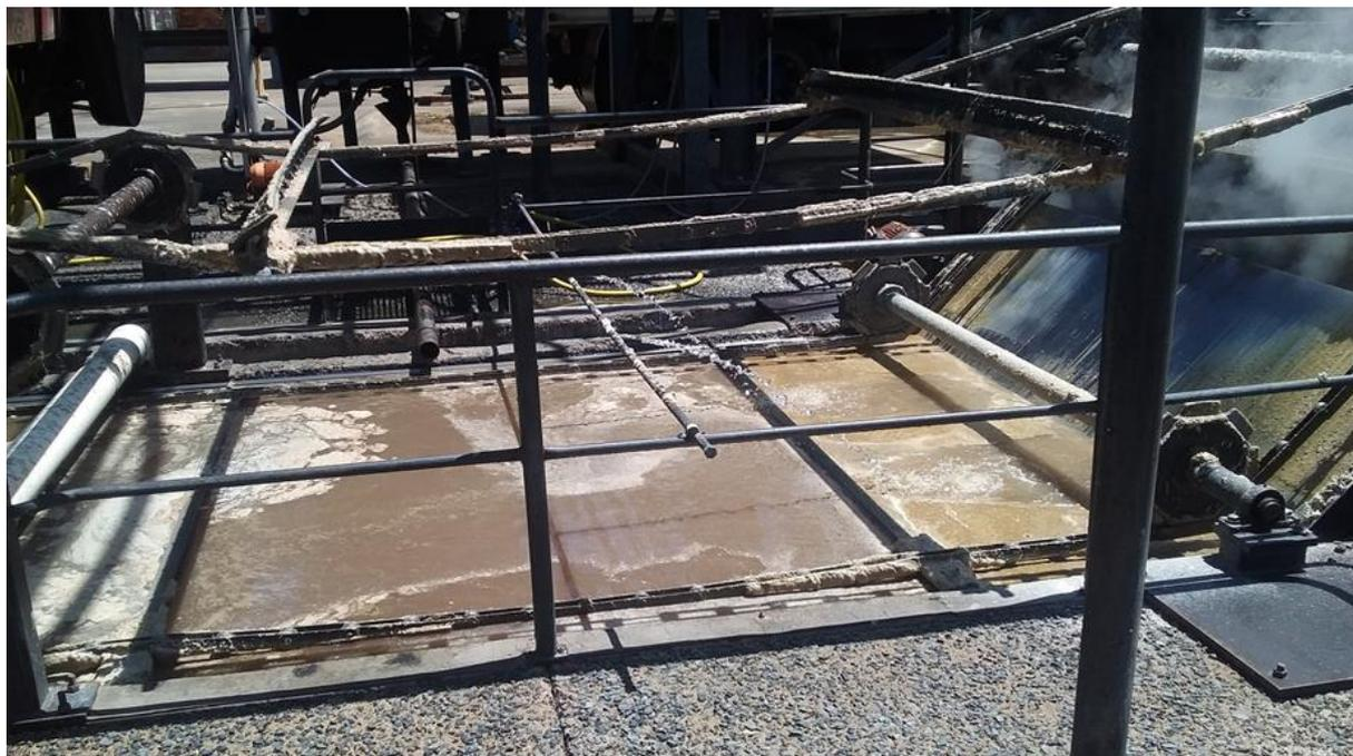
*Figure 30: DAF-saveall showing surface paddle scraping white to brownish beige surface FOG up an incline for dumping in the FOG separation and collection hopper*
