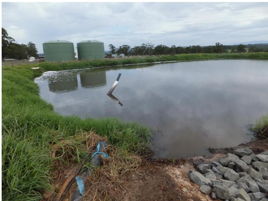
*Figure 7: Non-lined dam 3, which receives wastewater from dam 2 via gravity feed pipe seen here and with nearby reclaimed tanks in the background used for yard washdown and stone overflow channel to adjacent dam 4*
