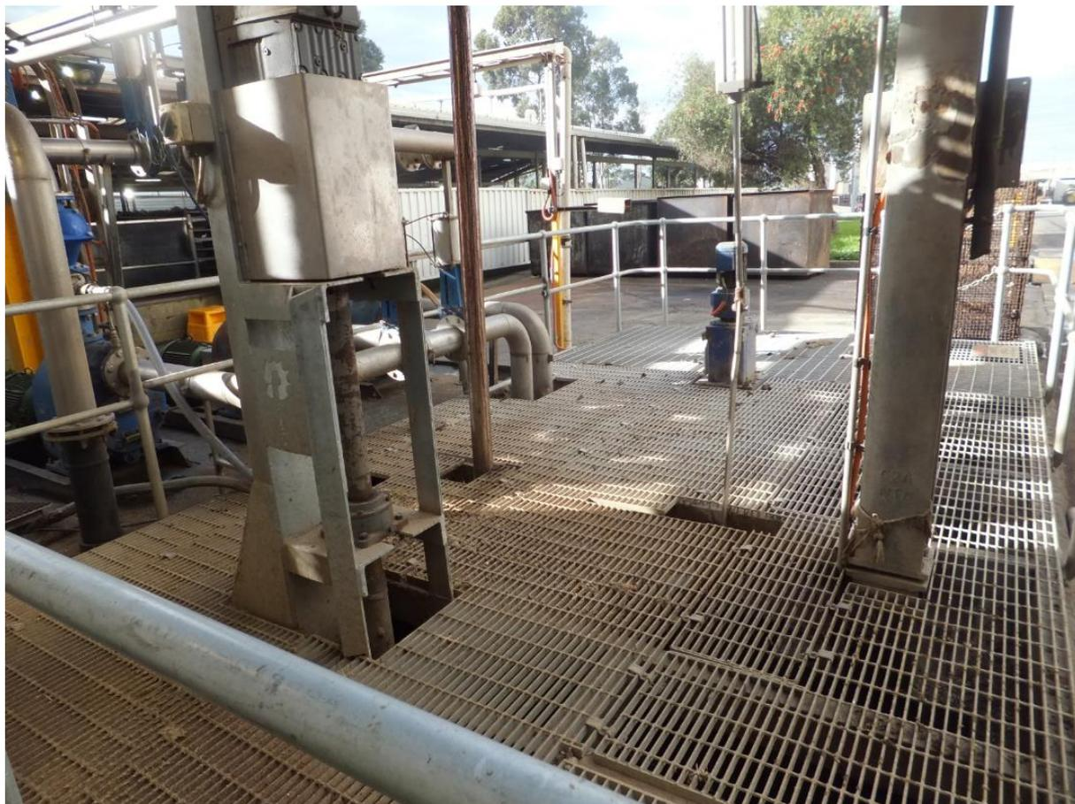
Figure 37: Adjacent Red and Green underground Pits with overhead mixing
