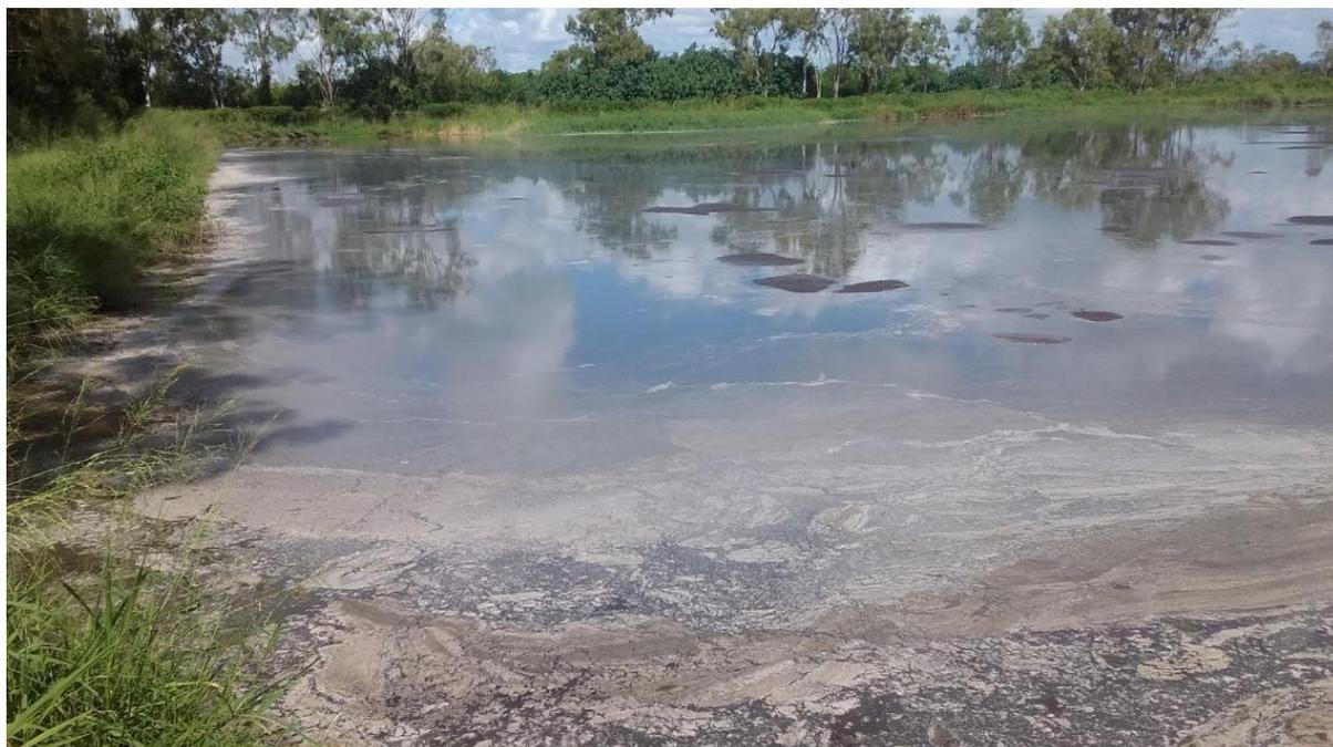
*Figure 32: Normal controlled processing with minor amounts of FOG passing through the DAF-saveall pit into around the edge of Dam 1*
