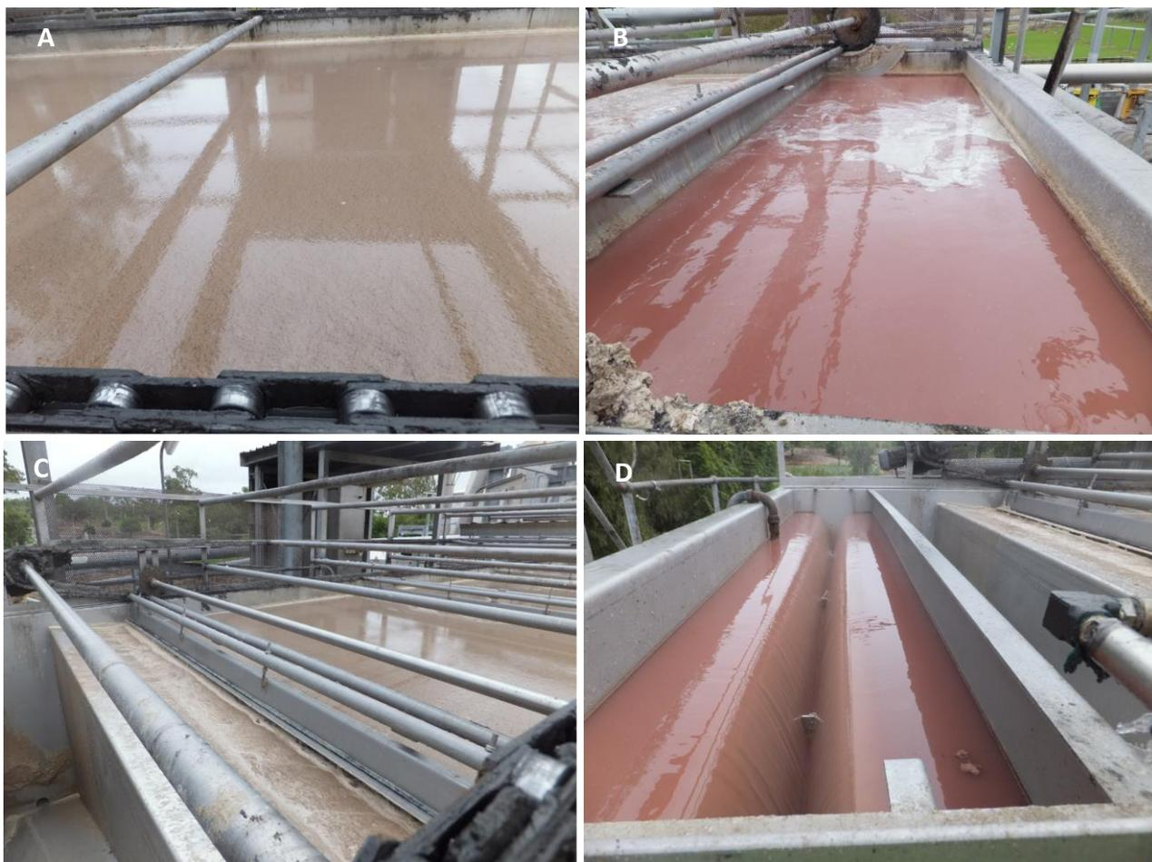
Figure 15: Dissolved air flotation (DAF) tank treating red stream wastewater, showing FOG flocculating (A), skimming off surface FOG (B), FOG collected separator tank (C, left) and separated red subsurface wastewater
