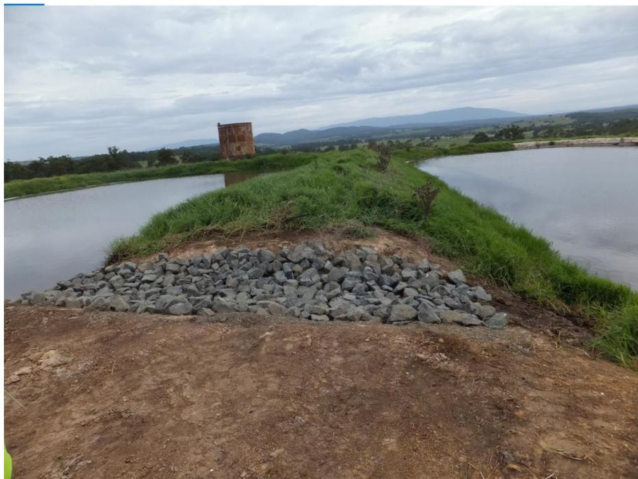
*Figure 8: Adjacent dam 3 (left) and 4 (right) connected via gravity feed 100mm PVC pipe showing a difference in elevation and stone overflow channel with the stormwater dam in the background for supplementing water in dam 3*
