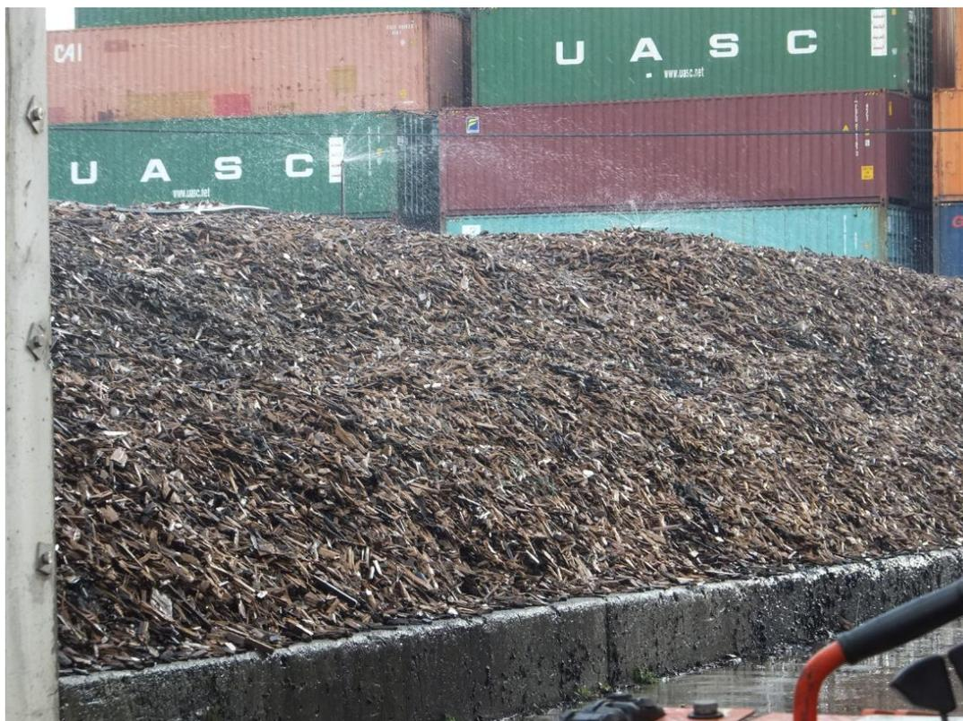
*Figure 36: Pine bark biofilter used to remove odorous air from the rendering plant which is pumped through the bottom with water sprinkling on the surface*
