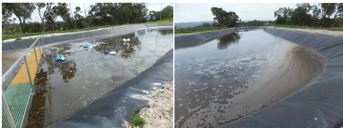
*Figure 4: Plastic lined dam 2 which receives wastewater from dam 1 via gravity feed pipes*
