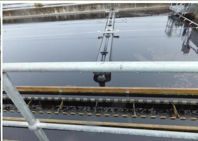
*Figure 19: Aerobic Biolac digester lagoon for biological nutrient removal (BNR) with variable aerated and non-aerated lanes (A), minor surface crusting on some edges and corners (B) and skimmer skimming flocks and weir for clarified water collection sent back to the BNR and clarifier (Figure 20)*
