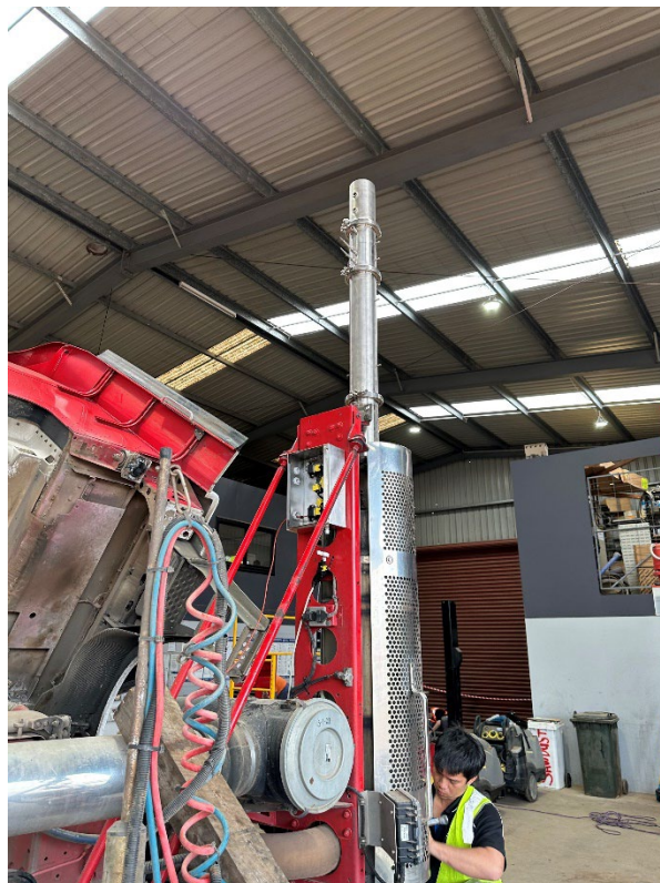
Figure 9: mini PEMS installation in progress.
