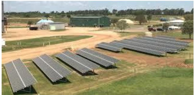
*Tracking ground-mounted solar PV systems* track the position of the sun on either 1-axis or 2-axis are becoming more common. Tracking systems produce more electricity per installed unit, but cost more to install. At feasibility stage a solar engineer will conduct screening analysis to determine whether a tracking system is viable.
