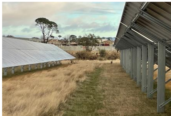
Figure 4: Panel-to-ground clearance (right of image above) and demonstrating dual land use.
