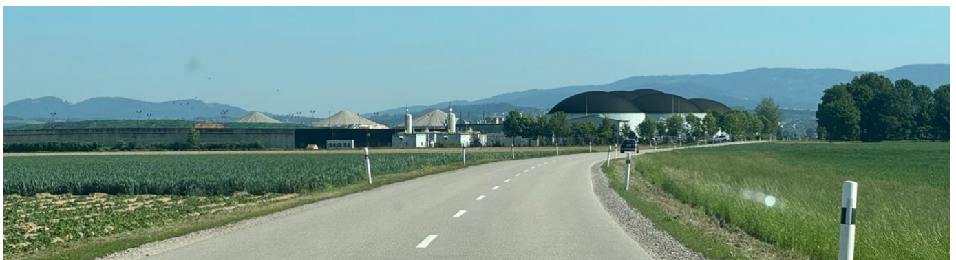
Figure 11. Outside view of Biomethane and Food Grade Bio-CO 2 Facility at Farming Operations - EON Aiterhofen.
