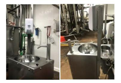
Simple bucket flow tests were performed, and savings were successfully gauged at around 70% with usage reducing from 7 l/min (existing) to 3 l/min. These results were significant, but reliability was yet to be proven with nay previous opportunities failing due to fouling.
