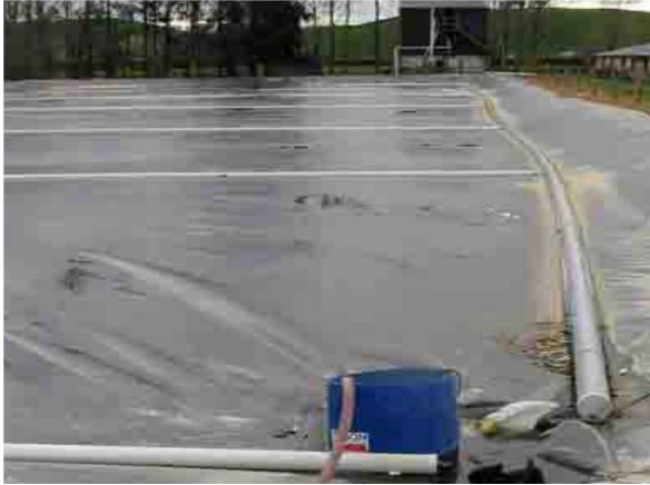
Figure 5 Weighed pipe and rainwater collection sump arrangement
