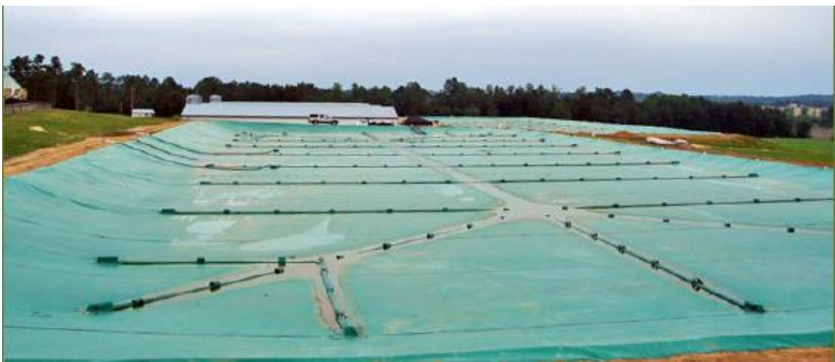
Figure 6 Covered anaerobic lagoon operating under a negative pressure gas collection system
