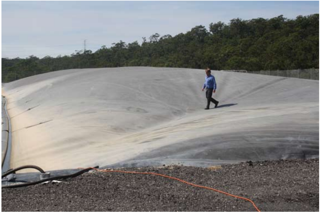
Figure 2: Covered anaerobic pond
