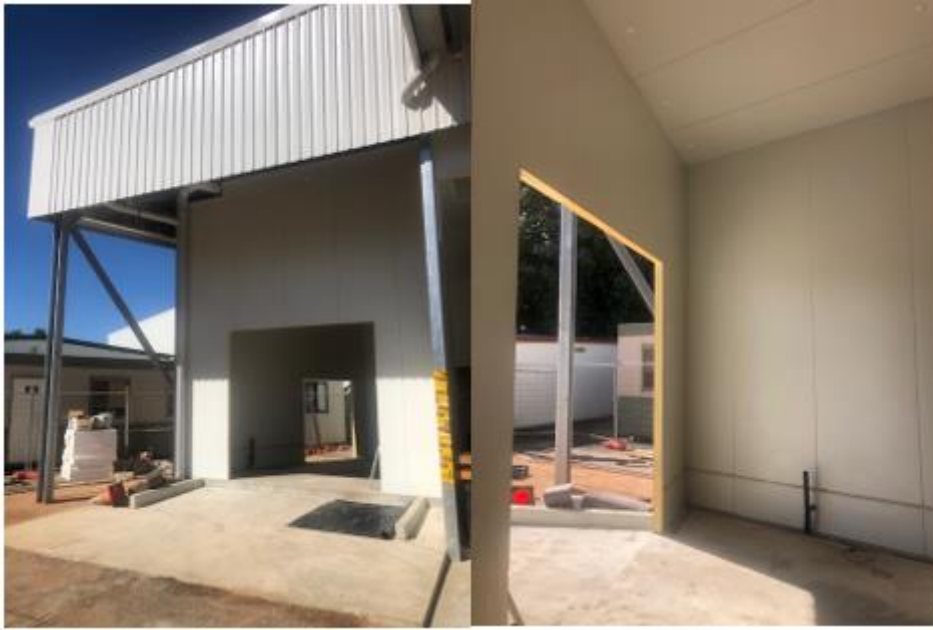
Image 1: Truck dock preparation for the Easi-Load / TRU-DOCK system.
