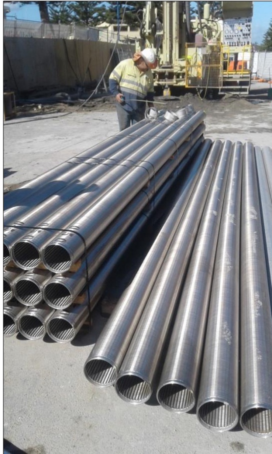
Figure 34: Lengths of slotted stainless-steel screen to be installed in a geothermal bore in Western Australia in 2017. Source: Rockwater Pty Ltd.
