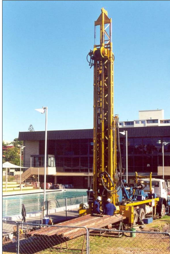
Figure 32: A rotary mud rig drilling at the Christ Church Grammar School geothermal project, Western Australia, 2001. Source: Rockwater Pty Ltd.
