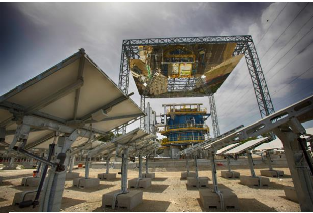
Figure 12: STEM tower technology (Magaldi)
