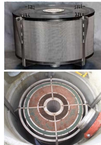
Figure 10: Ecosol filter with the StormDMT filter (Ecosol, 2017)
