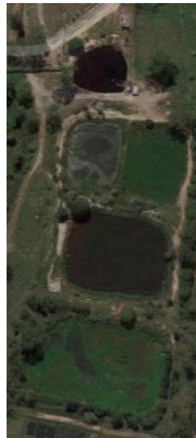
Figure 14: Decommissioned anaerobic ponds to treat stormwater runoff (to the south) and holding pond for treated runoff prior to release to sewer
