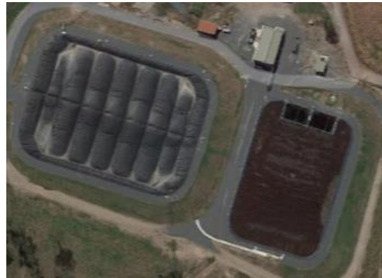
Figure 15: Site wastewater treatment system - covered anaerobic lagoon and Biolac® used for the removal of nitrogen.
