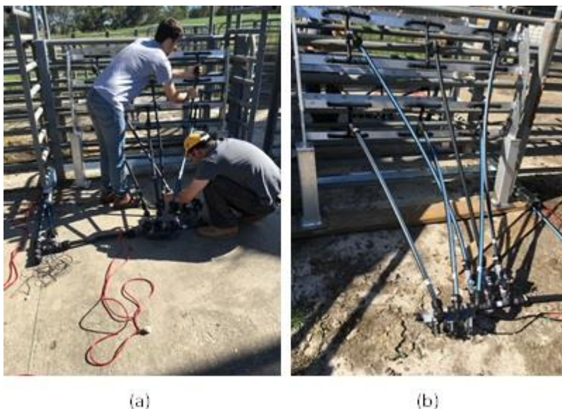
Figure 16. Assembled nozzle arrays on either side of the race way: (a) side A of the race way (b) side B of the race way.
