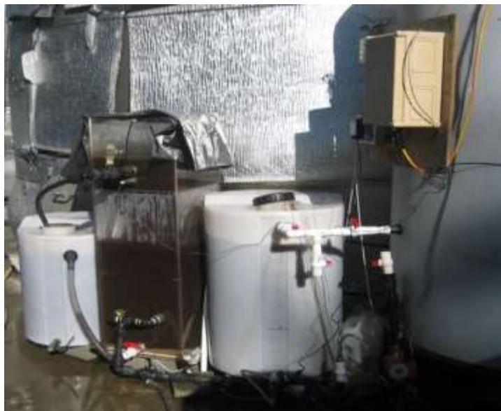
Figure 9: Struvite crystallisation plant installed at Site A to recover phosphorous from anaerobically digested paunch
