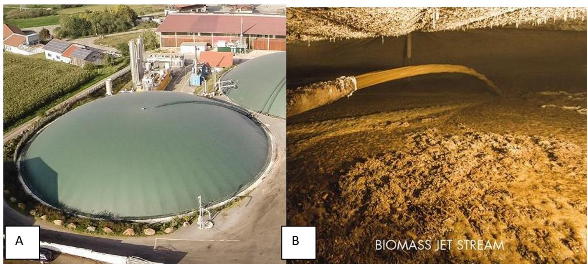
Figure 4: A) Anaerobic lagoon with double membrane roof and B) sprinkling nozzle (Sauter Biogas GmbH)
