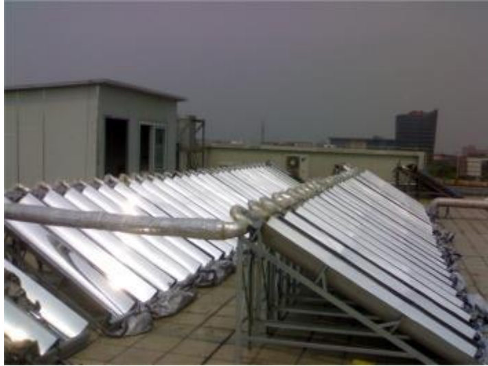
Figure 51 Photograph of the evacuated tube air heater [181]
