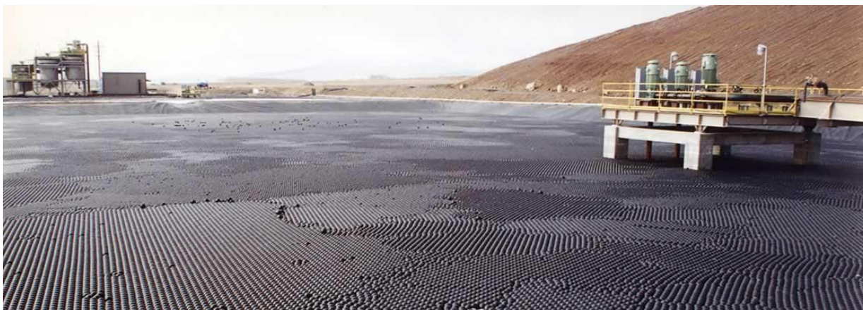
Figure 5: Image of a wind resistant floating pond covering 4 .
