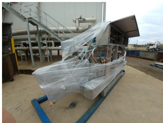
Figure 3-22 - Unloading at host site
