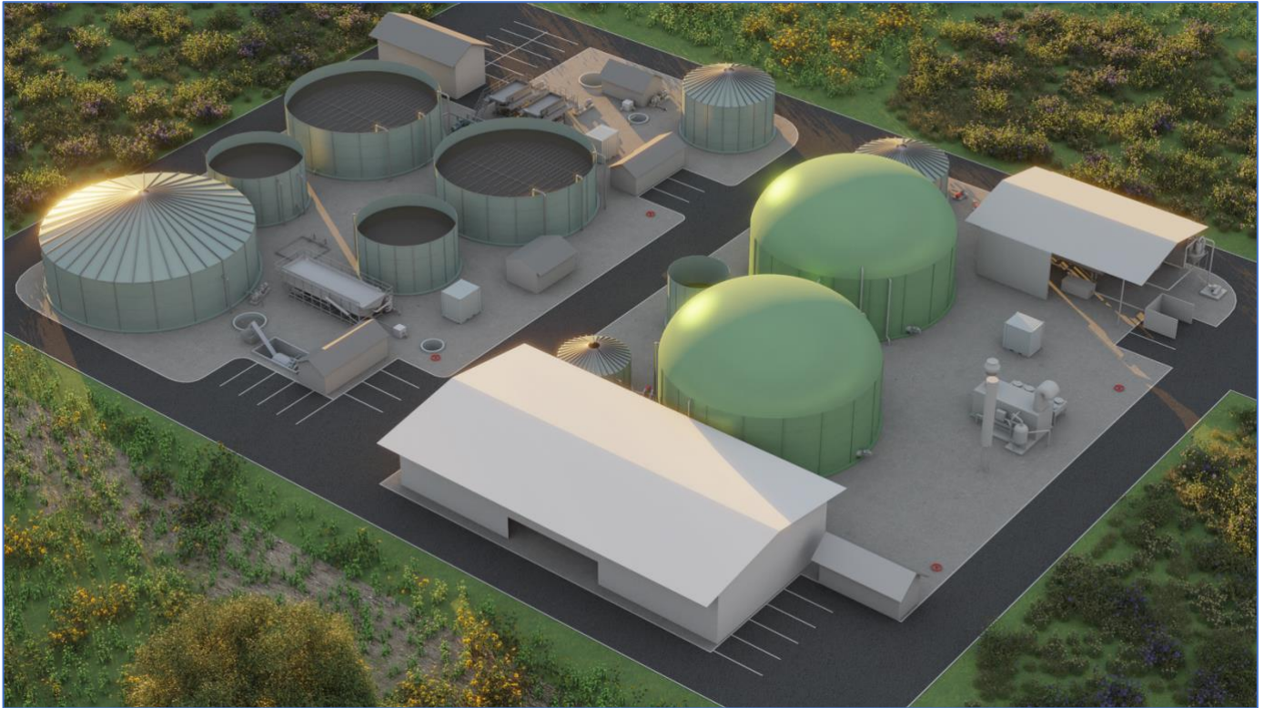
Figure 6. 3D Model of the Bio-Resource Recovery Facility, Including the Wastewater, Biogas and Biofertiliser Plants
