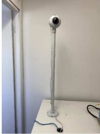
Figure 24- Installation of Overview Network Camera
