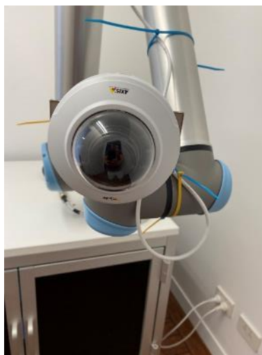
Figure 23- Installation of roll-face Network Camera
