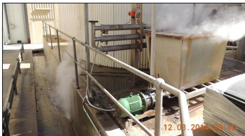
Steam-Trap passing large quantities of steam
