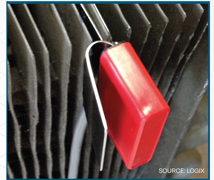
TEMPERATURE SENSOR ON EVAPORATOR
