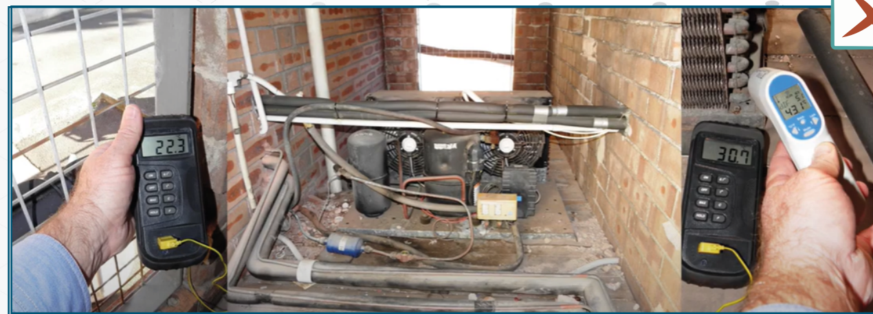
Inlet air temperature of 30.7 °C even though 22.3 °C fresh air is coming in from outside (+8.4 K increase!)
