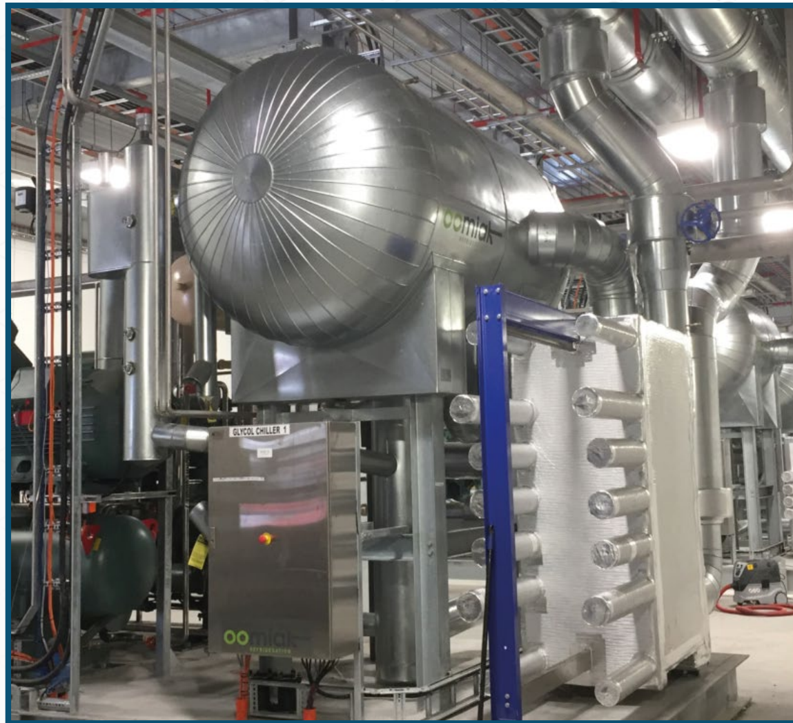
Ammonia/glycol systems in plant room
