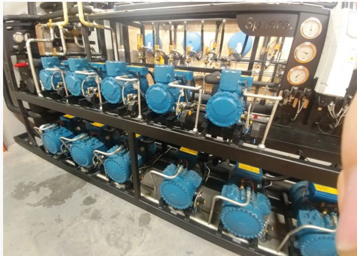
Full CO 2 system at NSW cold store, with transcritical (below) and low temperature compressors (above)
