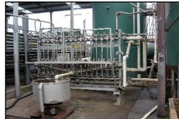
**Deoiling hydrocyclones** expel less dense oil and grease through the top of the unit while water flows out the base. This hydrocyclone requires very effective screening of the wastewater to minimise blockages and are generally most effective on non-render red streams.
