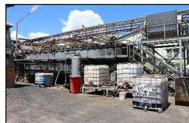
DAFs can be undosed or dosed. **Dosed DAFs** are more commonly applied in meat plants. The process is exactly the same except that chemical coagulants and polymer are mixed into the wastewater feed, increasing the removal of oil and grease, suspended solids and Chemical Oxygen Demand (COD).
